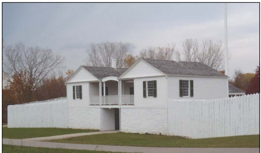
Restoration complete — the reproduction Commanding Officer's office (left) and the restored 1830s' guardhouse (right), both set on a new reproduction foundation that includes (on the lower level) jail cells and an interpretive room, surrounded by a reproduction wood stockade in its new location as part of Heritage Hill's Fort Howard complex. Photo by Nick Backhaus.
